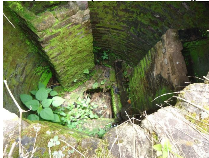
Figure 2: Inside the Gloss Kiln Chamber; build by Cardew note the back walls and the flue that leads to the bisque chamber. (Photo by Gukas 2016)
