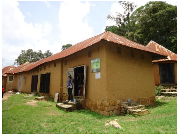
Figure 8: The Pottery Workshop centre now serves as a shopping center (Photo by Gukas 2016).
