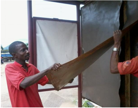
Plate X: Removal of inbuilt steel sheets Source: Researchers work, 2012
