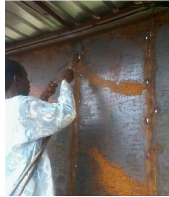
Plate XI: Welding of holes and hangs, Source: Researchers work, 2012
