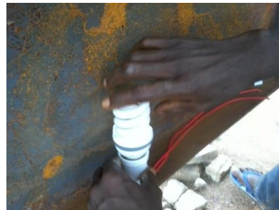
Plate XIII: Insertion of bulb into lamp holder Source: Researchers work, 2012
