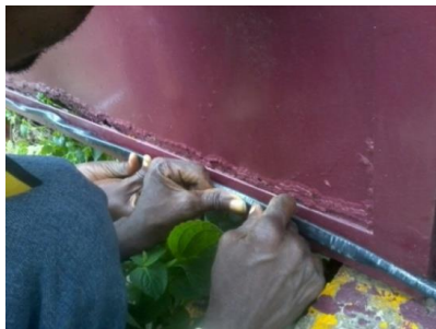
Plate XIV: Laying cables to the source Source: Researchers work, 2012
