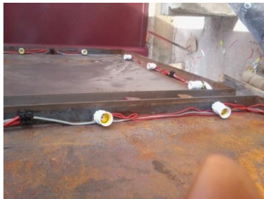
Plate XII: Cross section of wired lamp Holders and cables in the bus shelter Source: Researchers work, 2012
