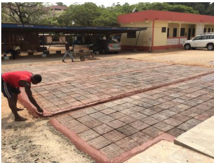
Plate I, Laying the recycled plastic-infused blocks. Source: NELPLAT
